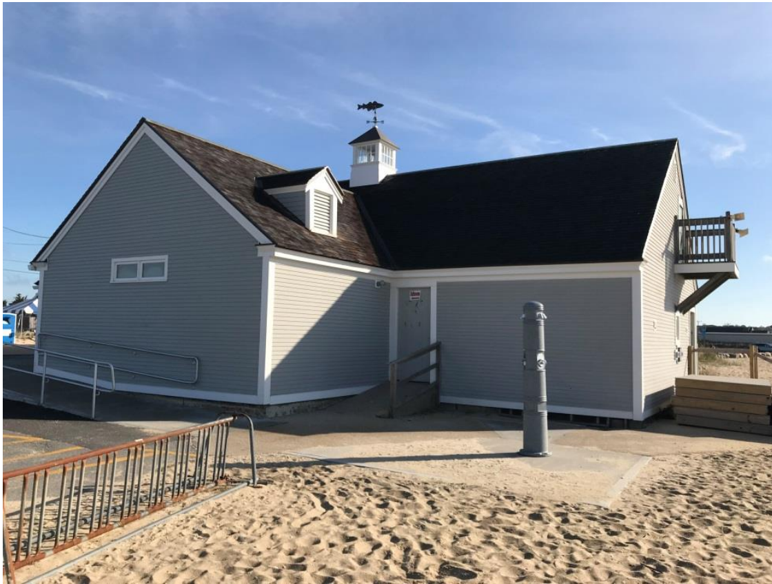
Craigville Bathhouse Septic Location
