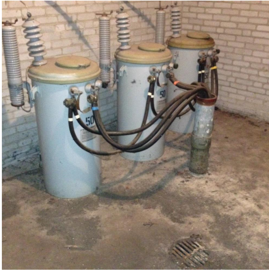
Typical Underground Transformer Vault
