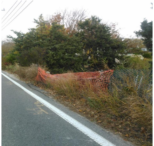
Snows Creek Culvert
