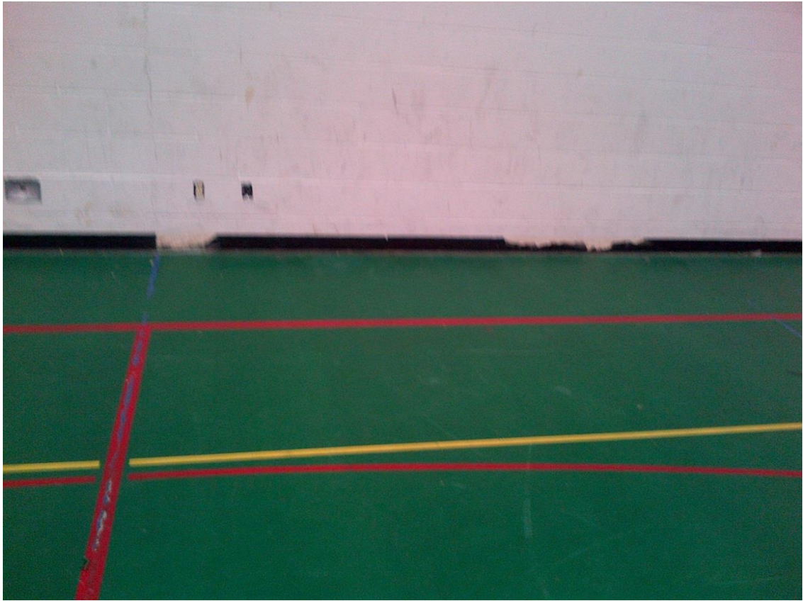
Barnstable High School Field House Floor
