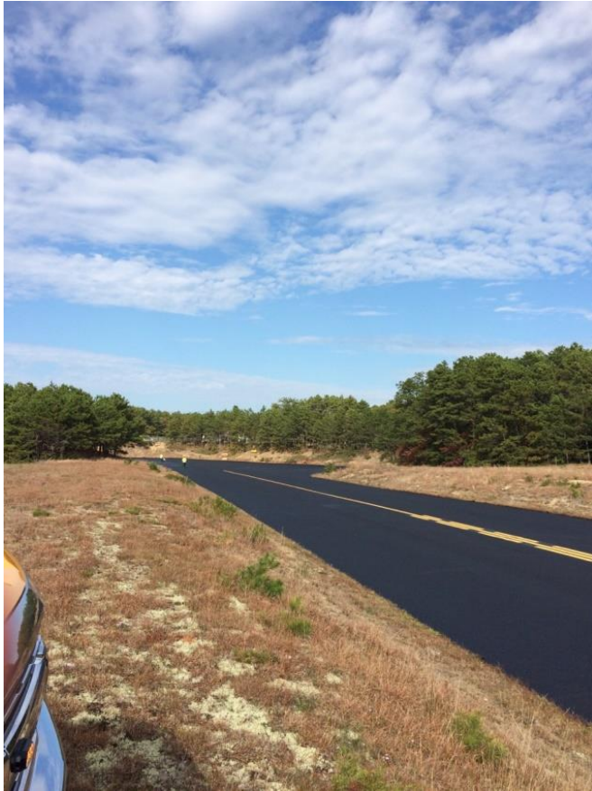
Runway 15-33 - Apply P-608 Surface Treatment and Repaint
