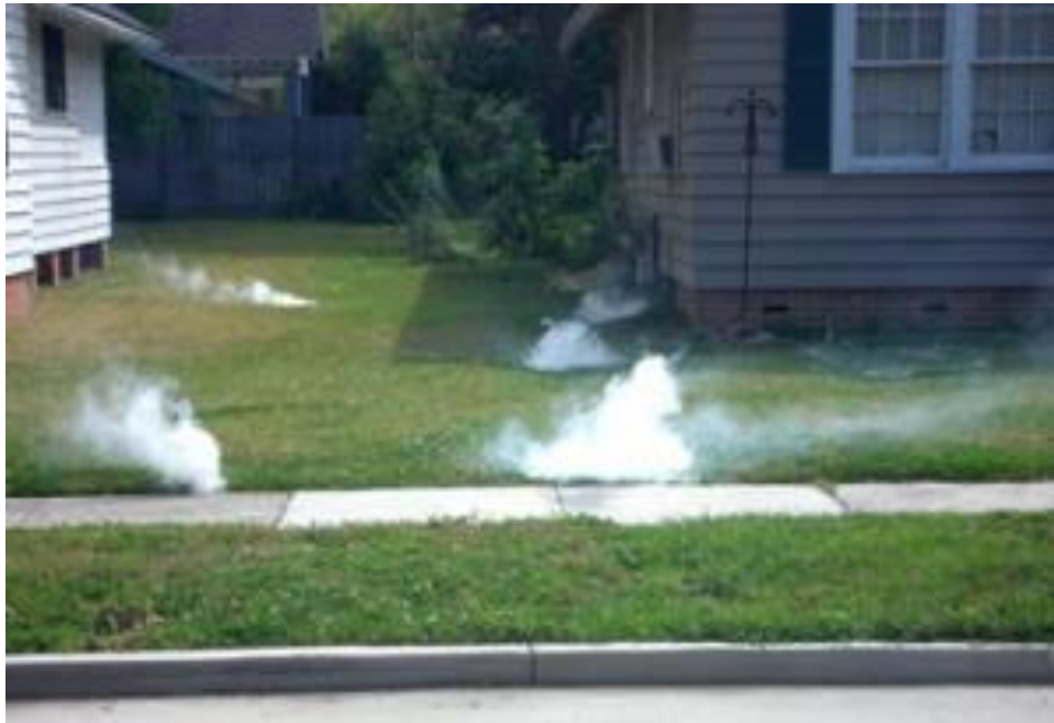
Sewer Smoke Testing
