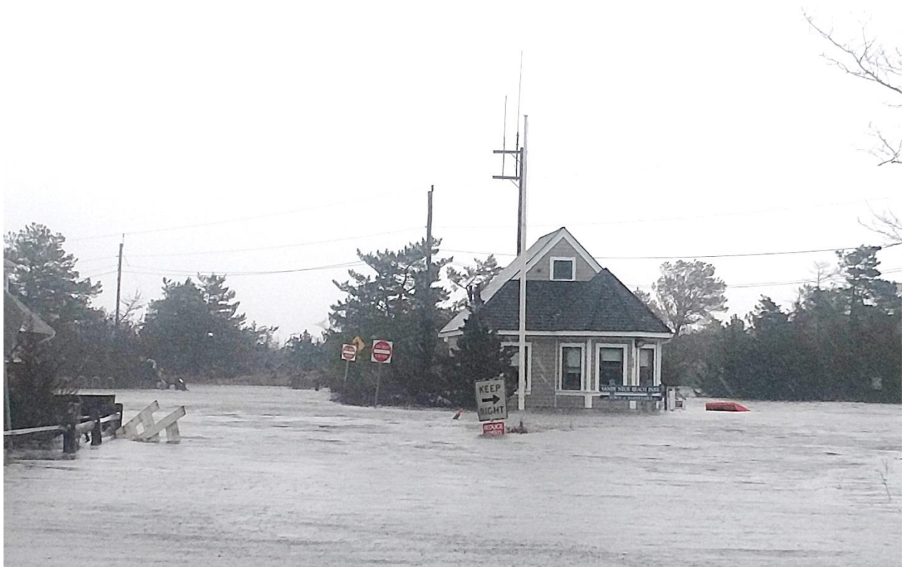
Sandy Neck Park Gatehouse Flood - 2018
