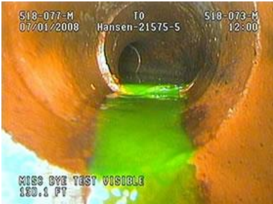
Sewer Dye Testing
